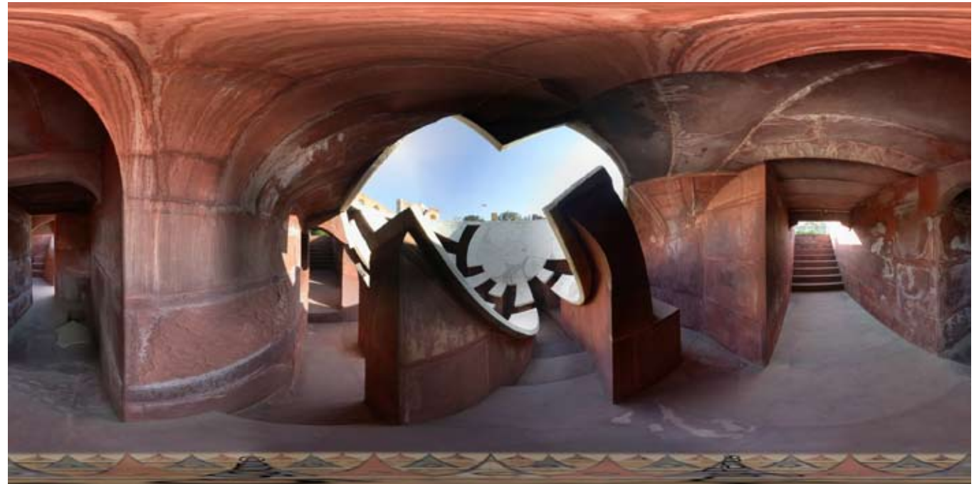
Panoramic view of the interior of the Jai Prakash at Jaipur. At far left is the passageway to the companion instrument, and at far right, exit steps to the outside. At center is the opening between hour segments of the hemispherical surface, with steps leading down to the center of the bowl.
