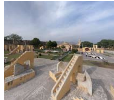
Two of the twelve instruments known as the Rasivalaya Yantras, foreground , at the Jaipur observatory. Each of the Rasivalayas refers to one of the signs of the zodiac, and is designed to directly measure the latitude and longitude of a celestial object at the moment that the sign to which it refers crosses the meridian.
